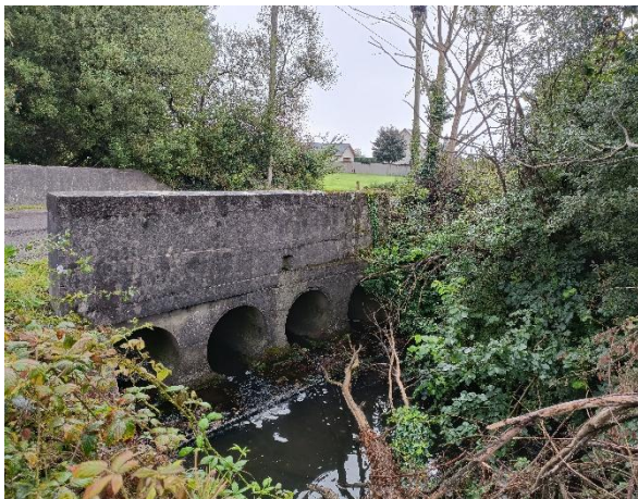
Plate 12A: Site LR11, view looking upstream showing quad-barrel culvert with flat concrete apron (23 Aug 2025)
