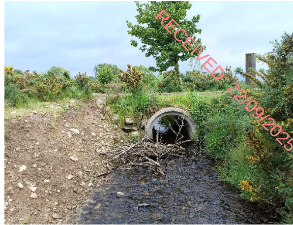
Plate 6B: Farm access culvert at Site LR6 with bare LHS bank upstream. Proposed cable undercrossing (17 May 2024)
