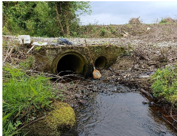
Plate 3B: Site LR3 culvert viewed downstream (17 May 2024)
