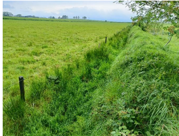
Plate 1B: Site LR1 upstream of local road (17 May 2024)
